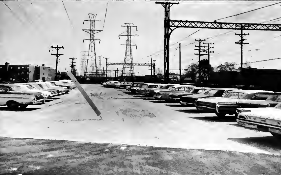
Enlargement work was undertaken within a few days and then repeated once. On May 4, 1964, when this photo was made, the need was so urgent that parking was permitted in this extension area even before construction was completed. Park'n'Ride space at this writing continues in short supply.
